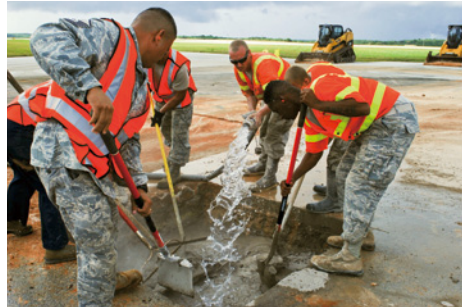
At Andersen AFB, airmen of the 38th Civil Engineering Squadron train in the latest airfield damage repair technique using rapid-setting concrete (January 23, 2014) (US Air Force photo/Airman 1st Class Emily A. Bradley)
